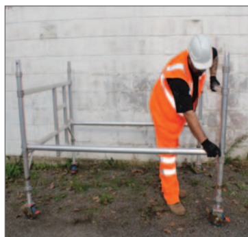
Leg adjustment and braked castor
