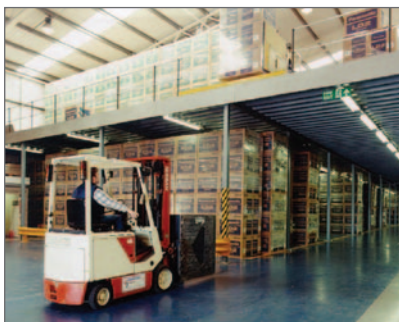
• Steel structural work incorporating a mezzanine floor
