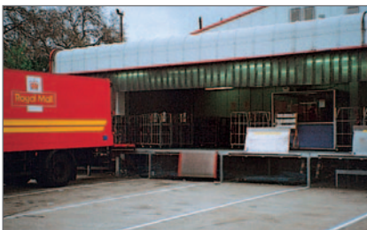
• Loading dock installation for the Royal Mail
